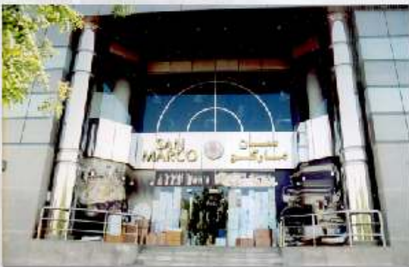
Column and Signages
