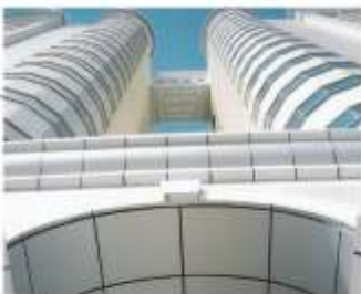
■ Soffits and Beams
